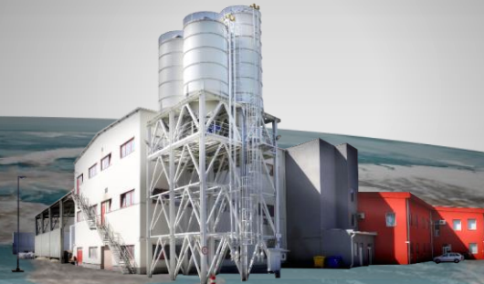
Plant-wide Smart Assets
